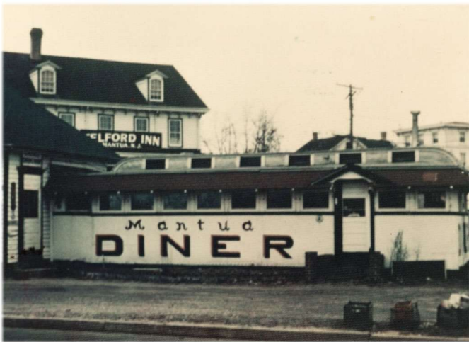
Mantua Diner, May 16, 1955, the Telford Inn is in the background.
