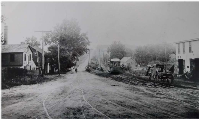
Looking North up Bridgeton Pike (Route 45) from the point at the Telford Inn
