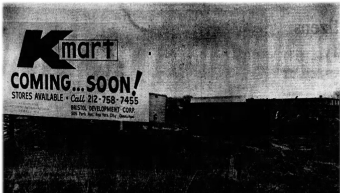
NEW K-MART shopping center being built on Route 45 near Berkely Road in Mantua will include an Acme supermarket and about 10 satellite stores. The 160,000 square-foot mart will open this spring. —Courier-Post Photo by John Avery
