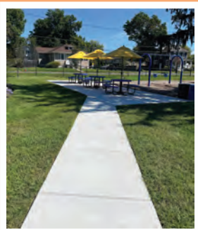
New concrete patio and sidewalk was added to McCarson Park
